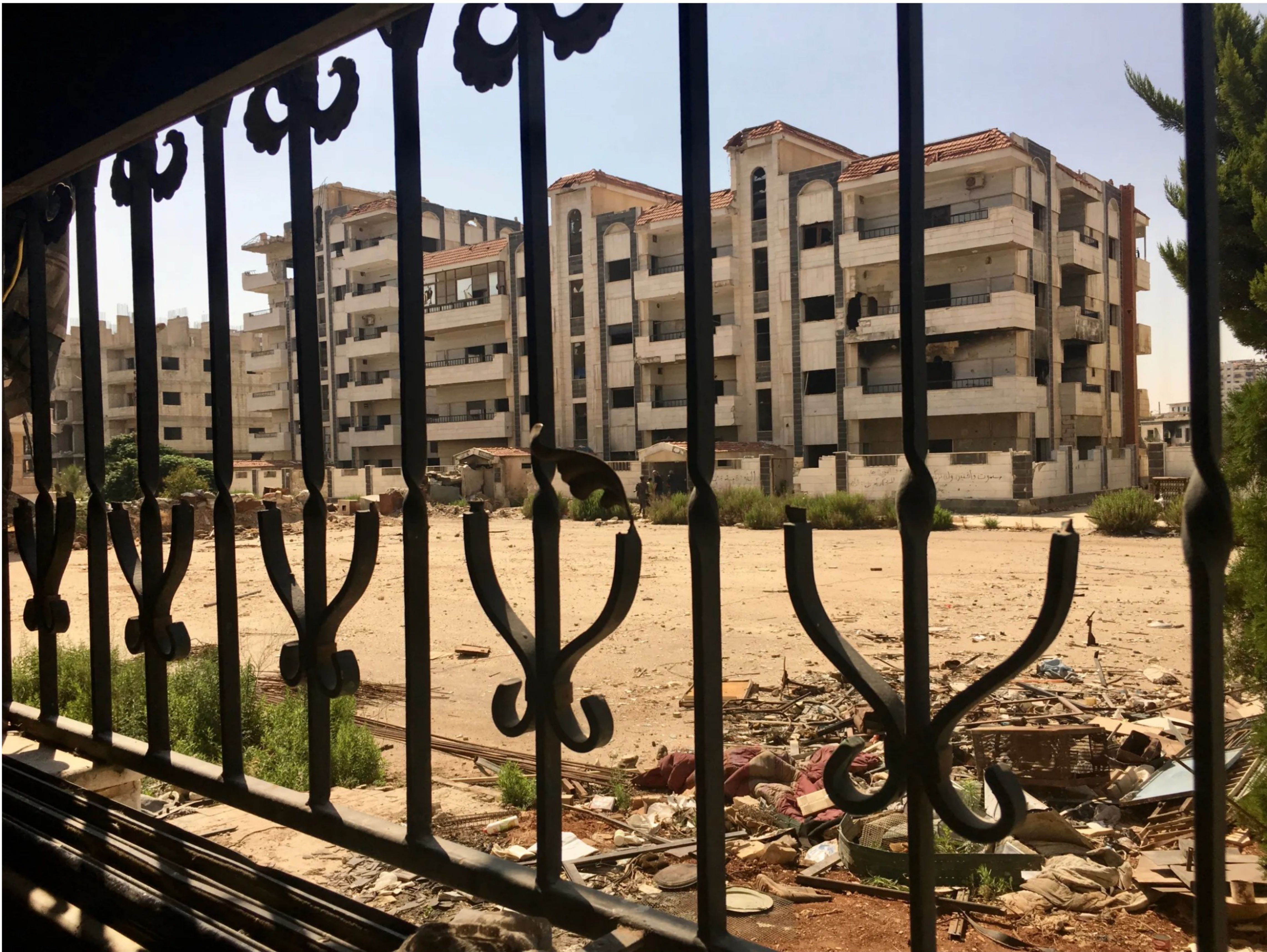
Damaged buildings in al Waer, a town on the outskirts of Homs in Syria
