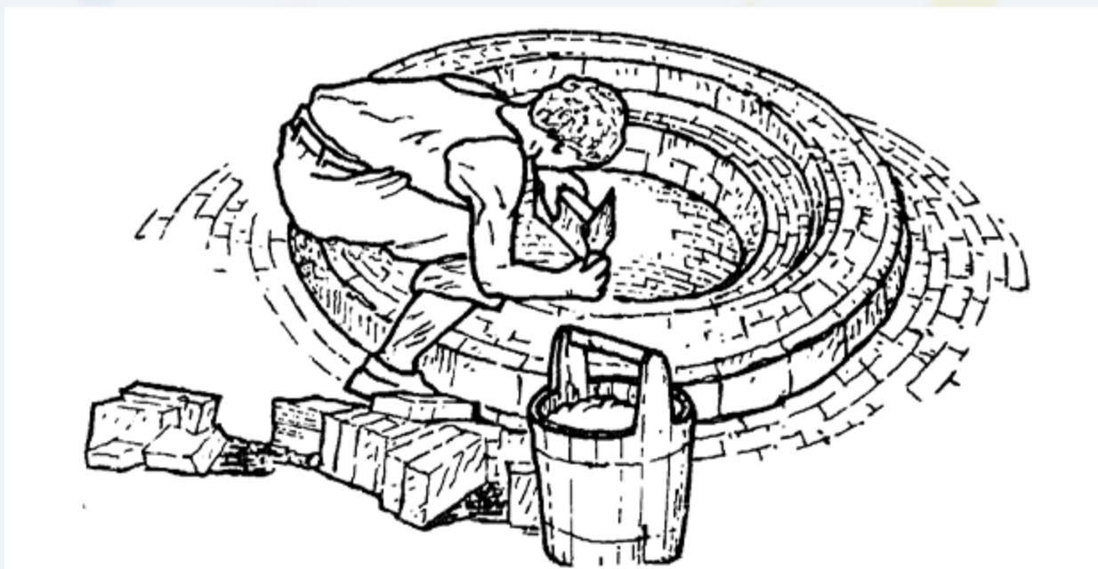
Fig. 4-12. Bricking the mouth of the pit without support.
